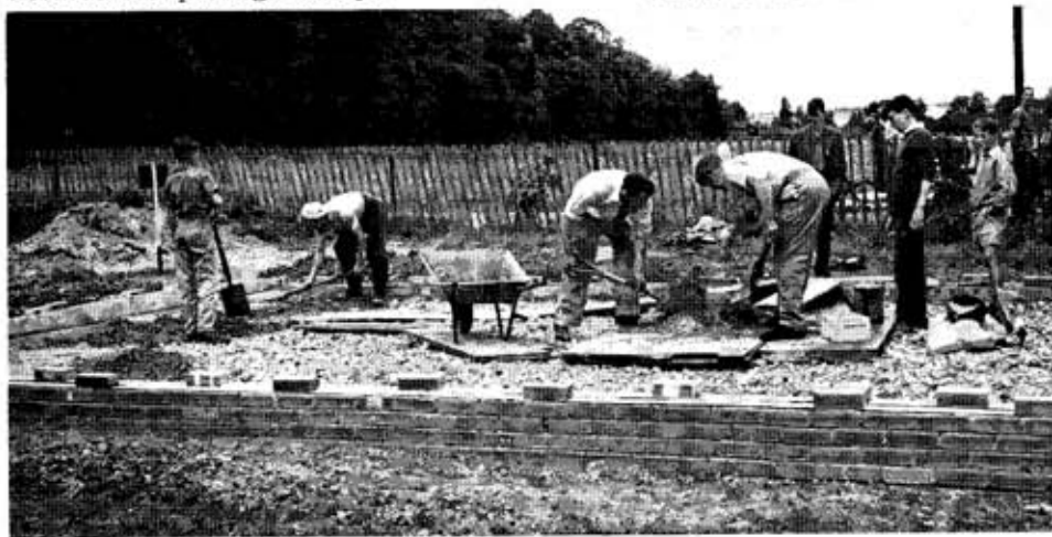
The Guildford clubhouse under construction in 1959.
