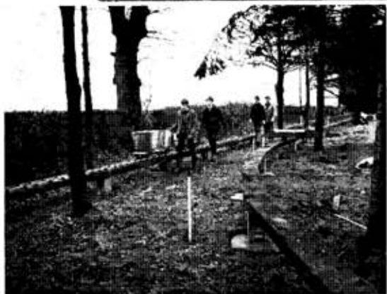
Above: Moulds and core-boxes are used for casting plinths for the high-level portion. Below: Loading a train to supply plinths and concrete to the railhead.
