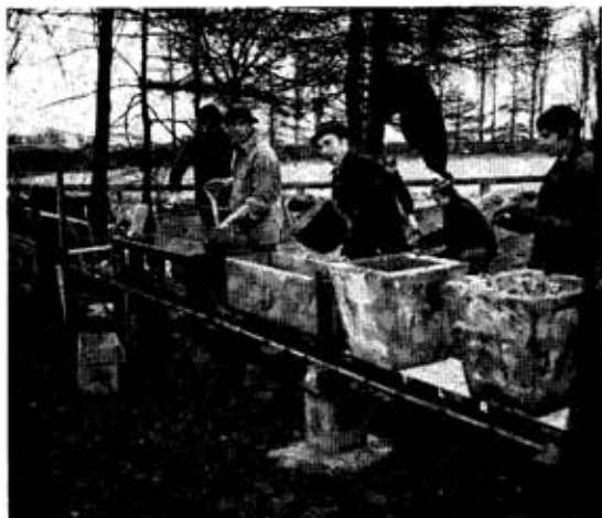
Above: Moulds and core-boxes are used for casting plinths for the high-level portion. Below: Loading a train to supply plinths and concrete to the railhead.
