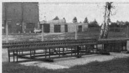
The double traverser.
