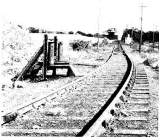
Rounding the bends: On the upper incline, entering the semi-circle. Note the de-railing switch.
